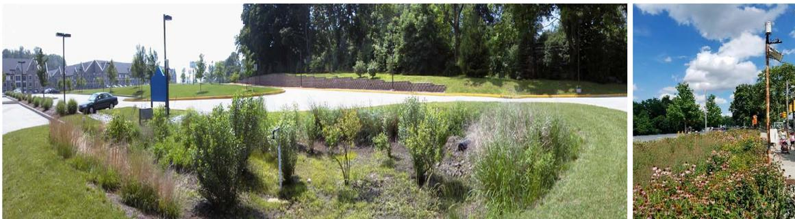
Figure 1. Bio-infiltration basins (left) Villanova and (right) Philadelphia.
