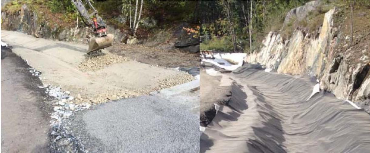
Construction of stream-bed and sealing of the stream-bed (FDP-membrane), Julsbekken project
